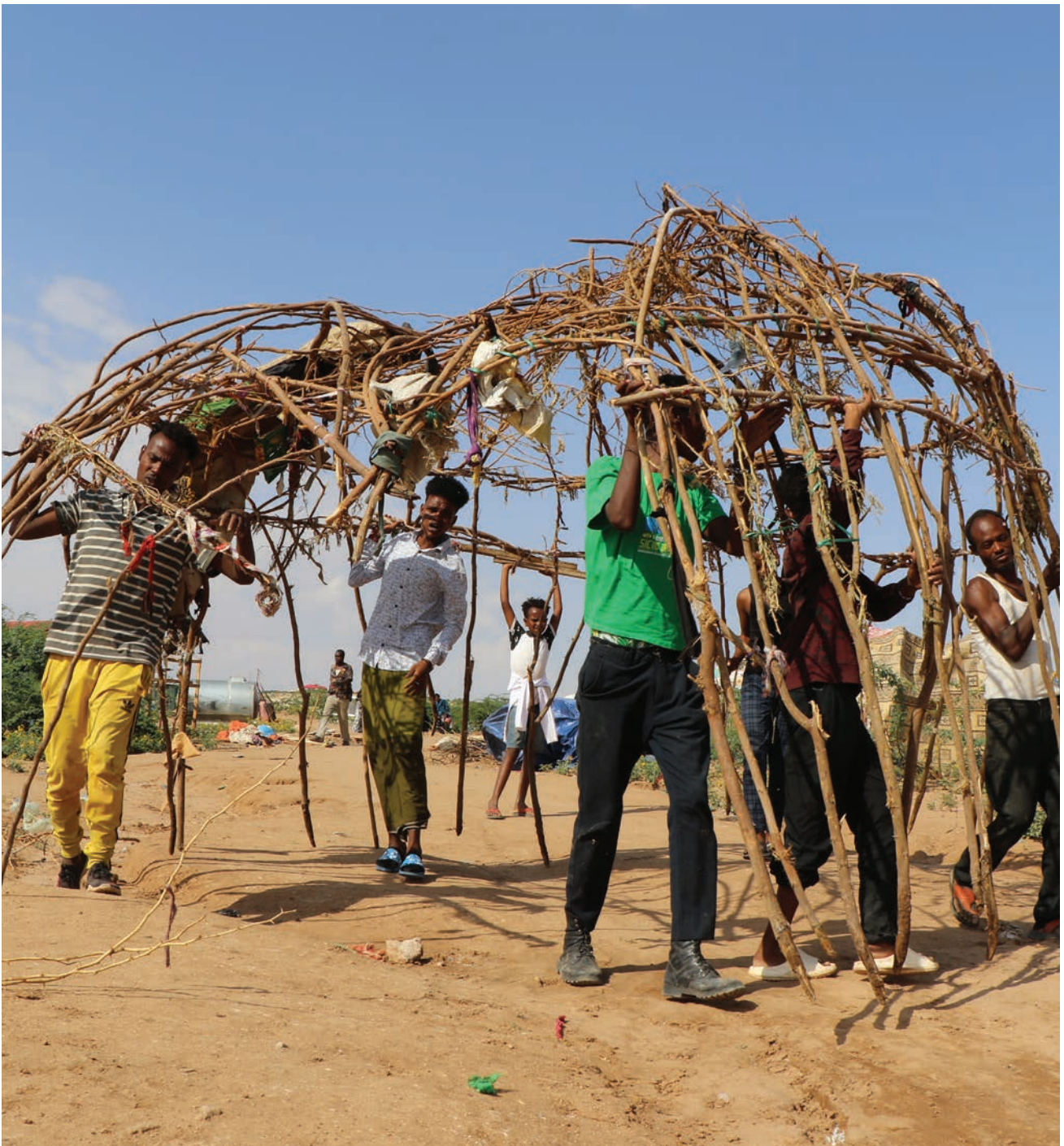
Group of men constructing a shelter structure
