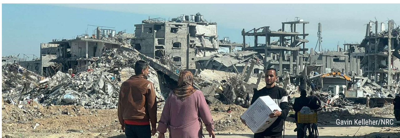
WIDESPREAD DESTRUCTION OF HOMES AND INFRASTRUCTURE IN BEIT HANOUN, NORTH GAZA
