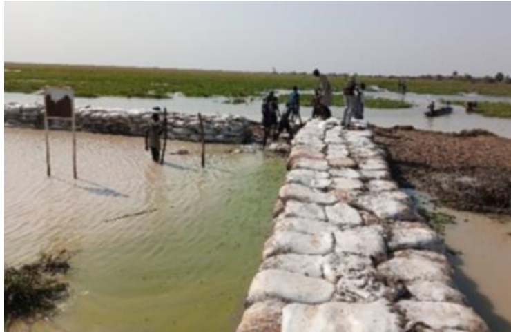
A rehabilitated flood control dyke at Ganyiel Payam, IRC cash for work programme. Photo: IRC
