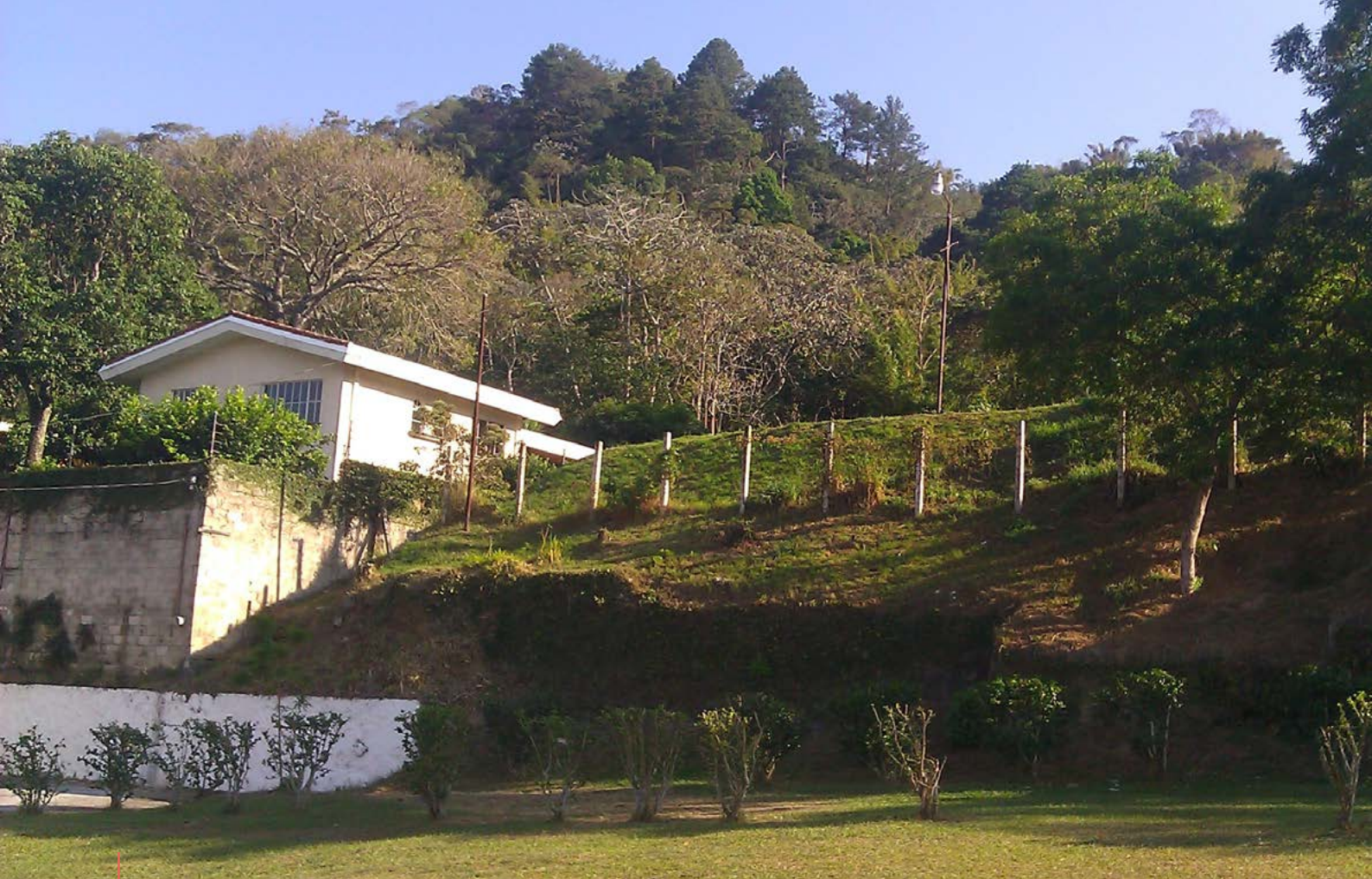
A house remains next to the scar of a major 2001 landslide in Santa Tecla. The residents apparently refuse to relocate in spite of the risks. Photo © Jeremy Harkey
