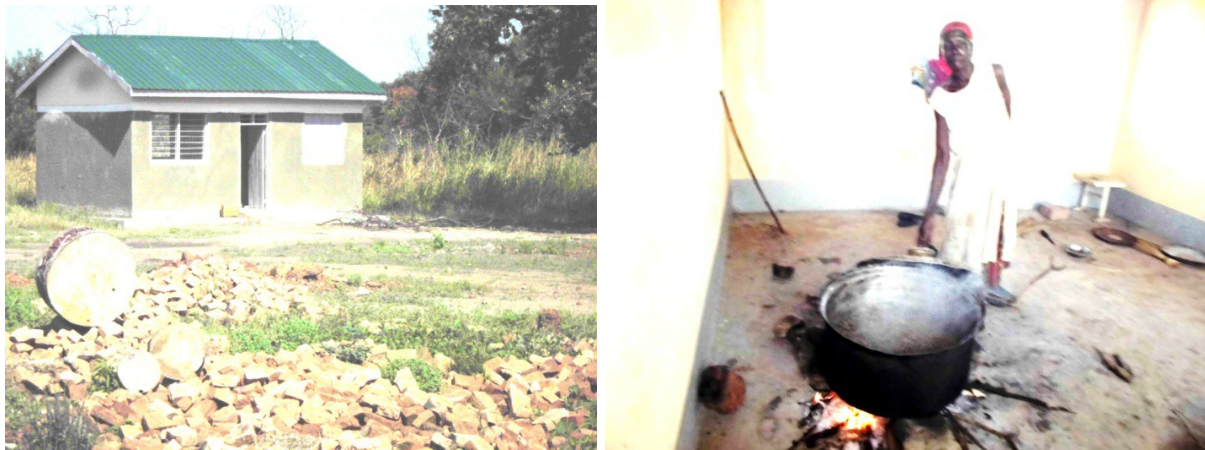
Figure 7: Kitchen/Storage (left) and Cooking stove on the floor (right) in Warahel Primary school. Floor based cooking is likely to lead to cracking, does not provide smoke ventilation and uses significantly more fuel than a stove. Photo: J. Makongo
