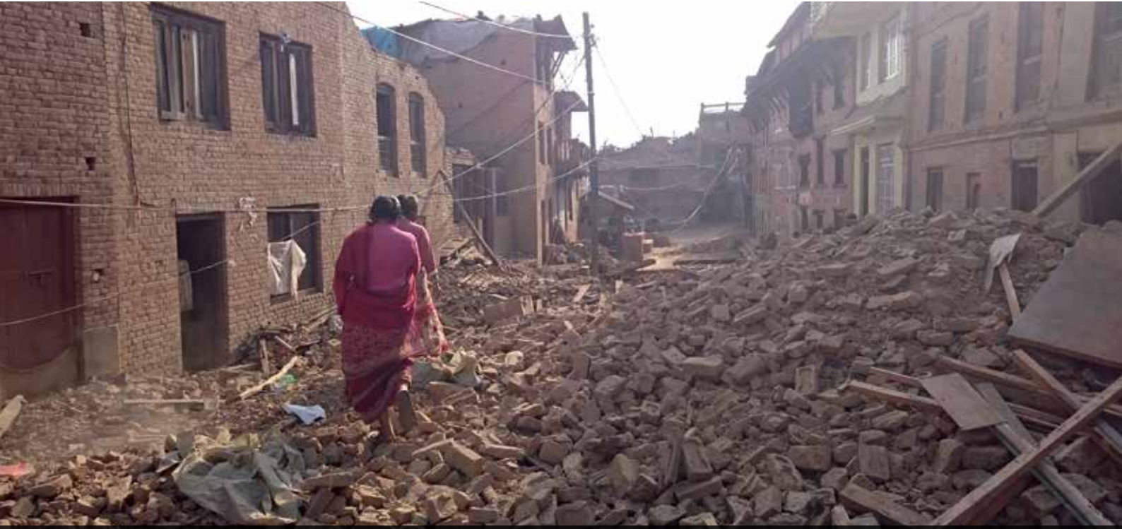
People walking in the streets surrounded by destroyed buildings, Nepal 2015. Photo: NRC/Per-Erik Stafanson.
