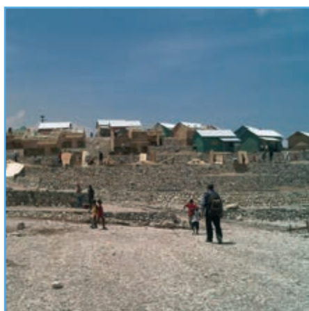
The Villambetta relocation settlement under construction. Photo: Havard Breivik/NRC
