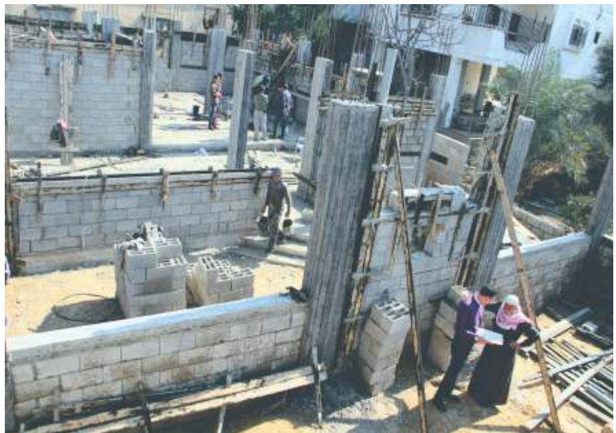
Construction site, Gaza Strip, 2013. Photo: NRC.
